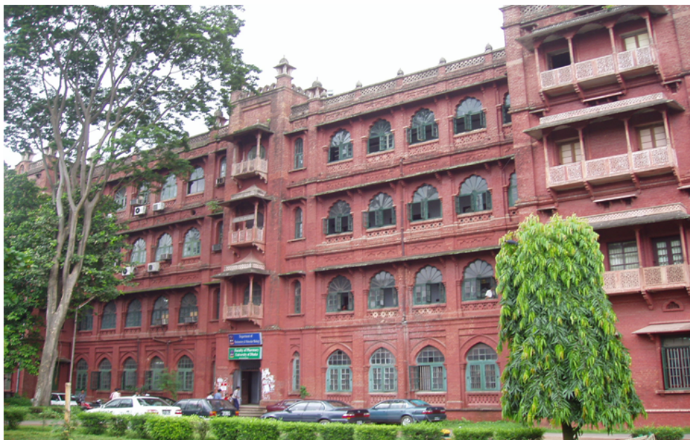
The old building in Curzon Hall area of the University of Dhaka, where the Department of Pharmacy started its journey in 1964. Presently, the office of the Dean of the faculty is situated in the ground floor of this building.
